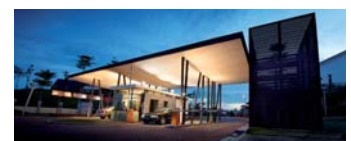
Tight security at East Ledang
